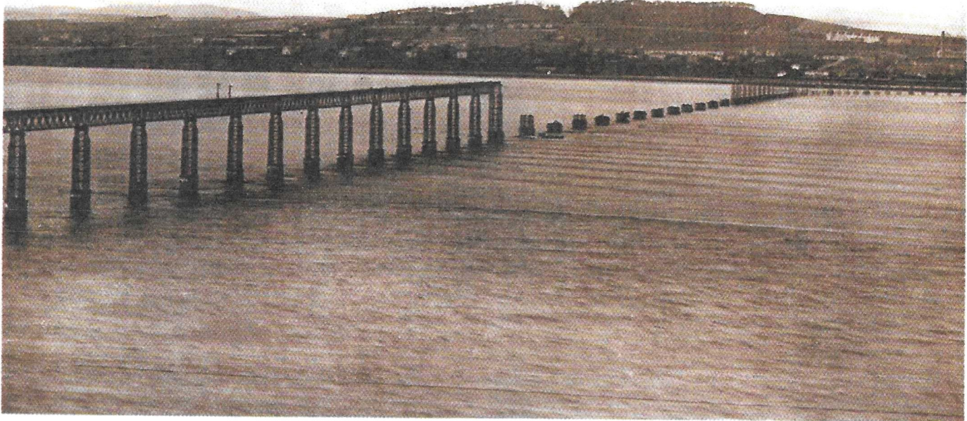
Fig. 4. Tay rail bridge after 1878 collapse (viewed from south)
