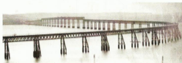
Figure 1. The original bridge
